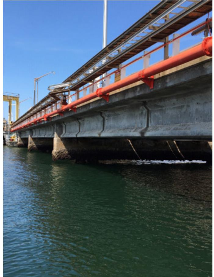
"Because of the low currents required to meet the prestressed steel and hazardous area limitations, the hybrid CP system required an initial power-up phase of three to four months before the external power source was disconnected and the system left to operate galvanically," explained David Celine, managing director of Omniflex. "The system comprises of nearly 35,000 embedded hybrid anodes that were installed
